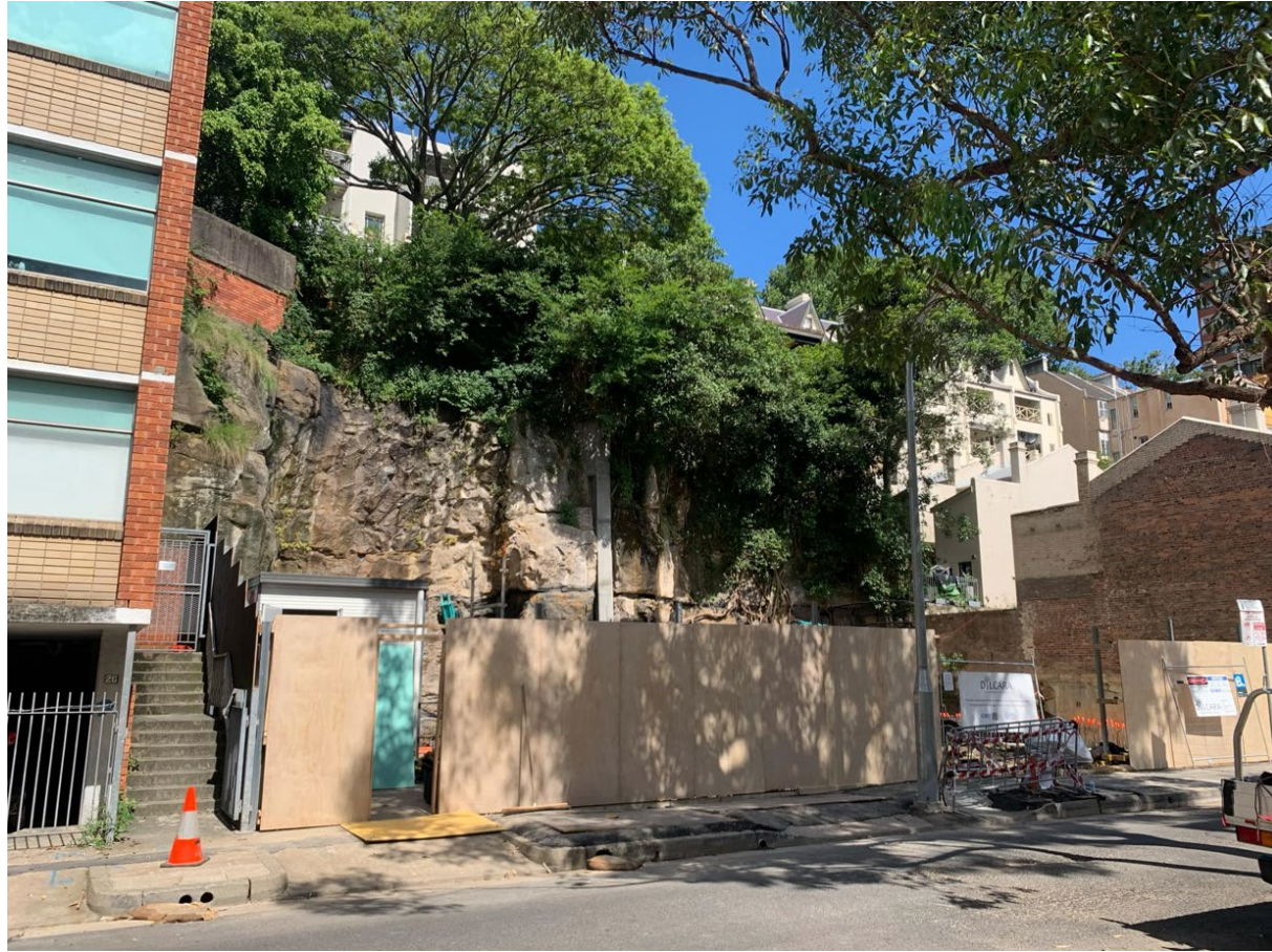
30A – 34 Brougham Street to south
